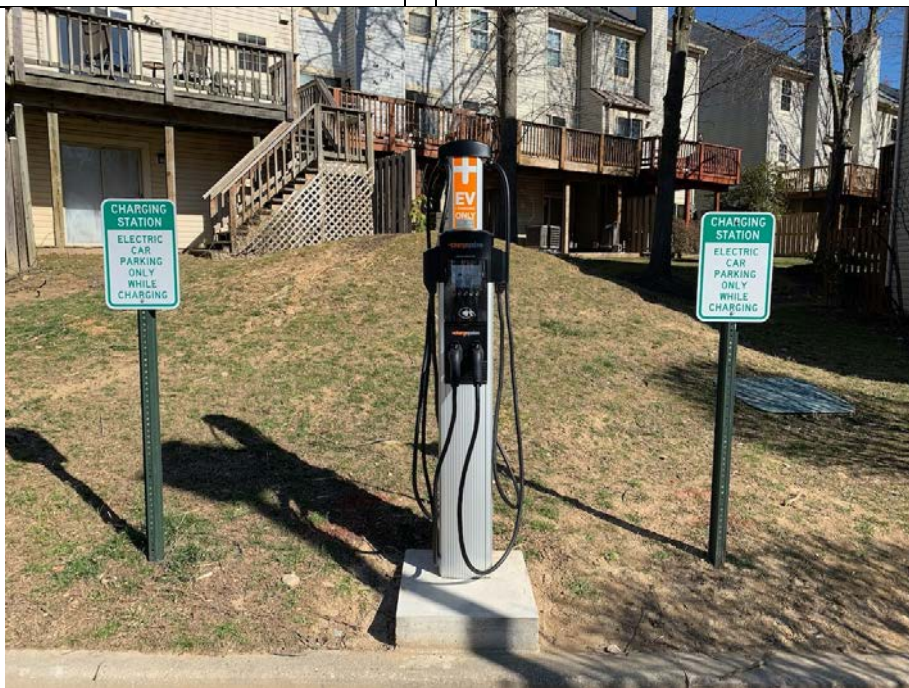
The station after installation and final inspection.
